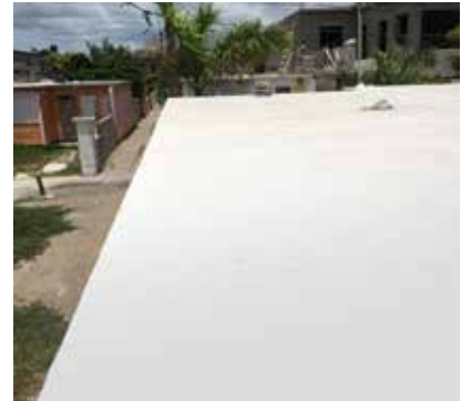
Fig. 5. Finished roof with 3 coats of Sikalastic®-560.
