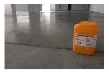
The expansion floor joints were sealed with **Sikaflex®-11 FC**+, a 1-component elastic polyurethane sealant.
